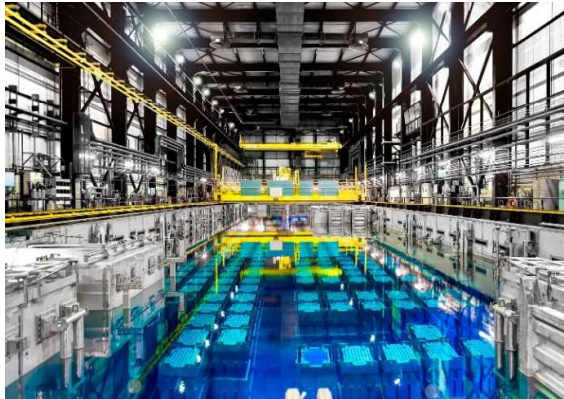
(a) Wet storage at the Orano reprocessing facility in La Hague, France
