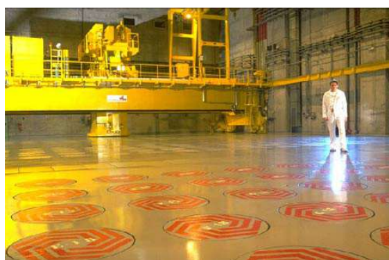
(b) Vitrified waste interim storage room
