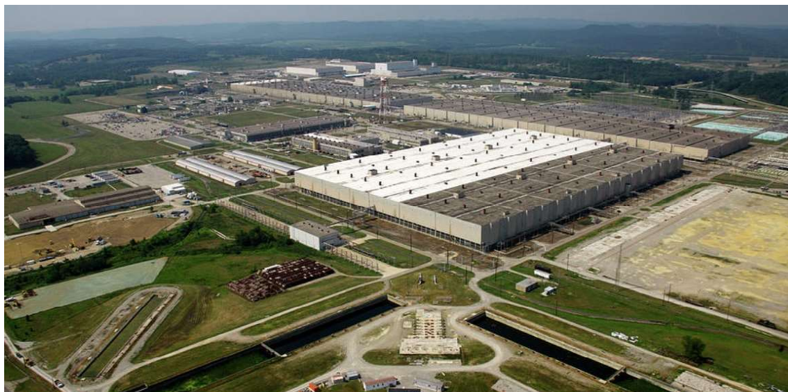
Figure 3.3.3-4. View of the Portsmouth gaseous diffusion uranium enrichment plant
