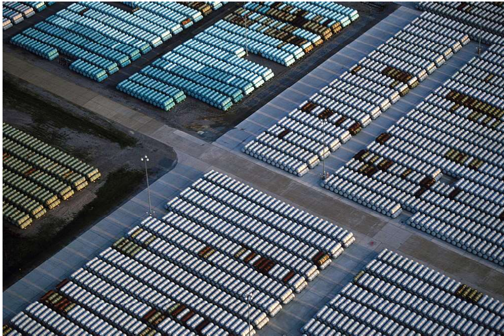
Figure 3.3.3-9. Aerial view of the depleted UF_6 cylinder storage yard at the Paducah gaseous diffusion plant (USA), storing about 38 000 used cylinders in 2001
