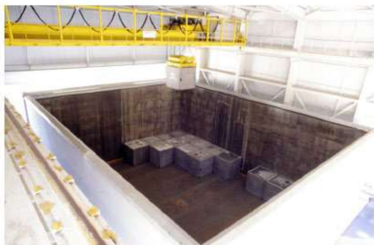
Figure 5.1-5. El Cabril near surface disposal facility, Spain.
