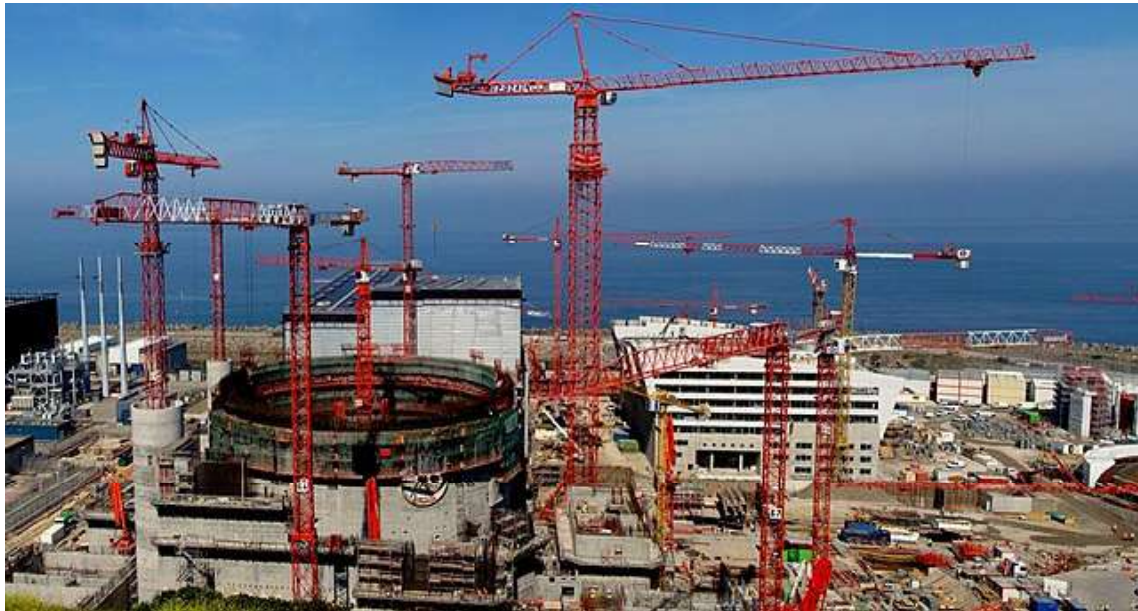
Figure 3.3.7-1. Unit 3 of Flamanville NPP under construction (France, 2010)
