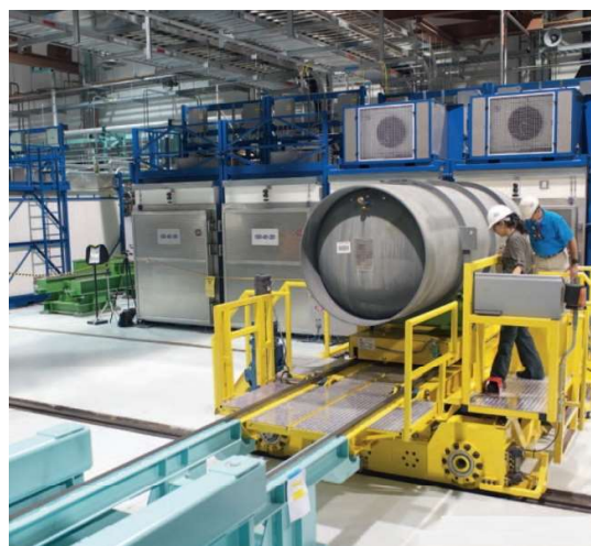
Figure 3.3.3-2. A transport cylinder is prepared for handling at the plant
