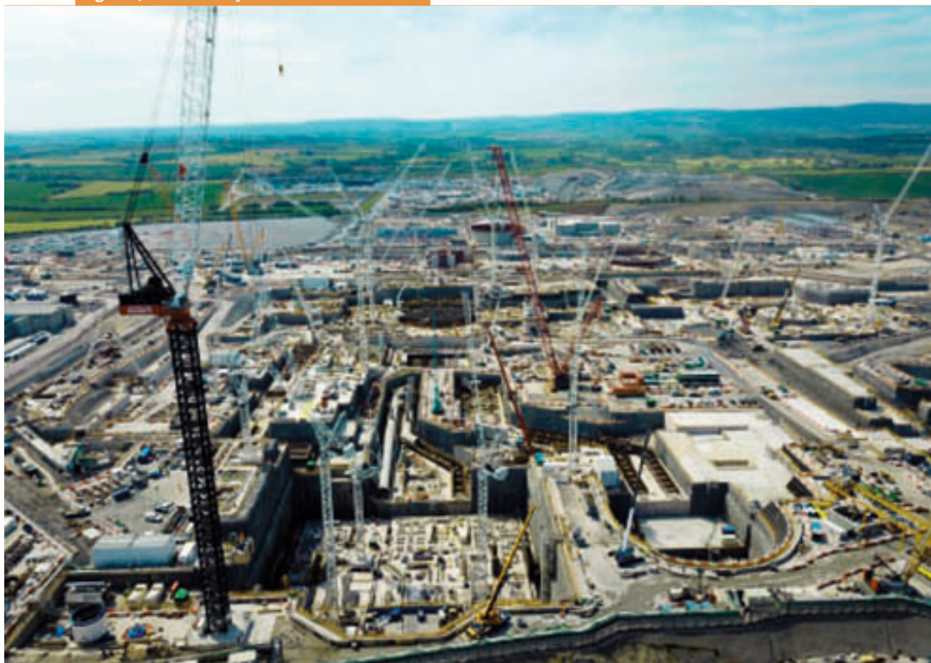
Figure 42 - The Hinkley Point C Construction Site
