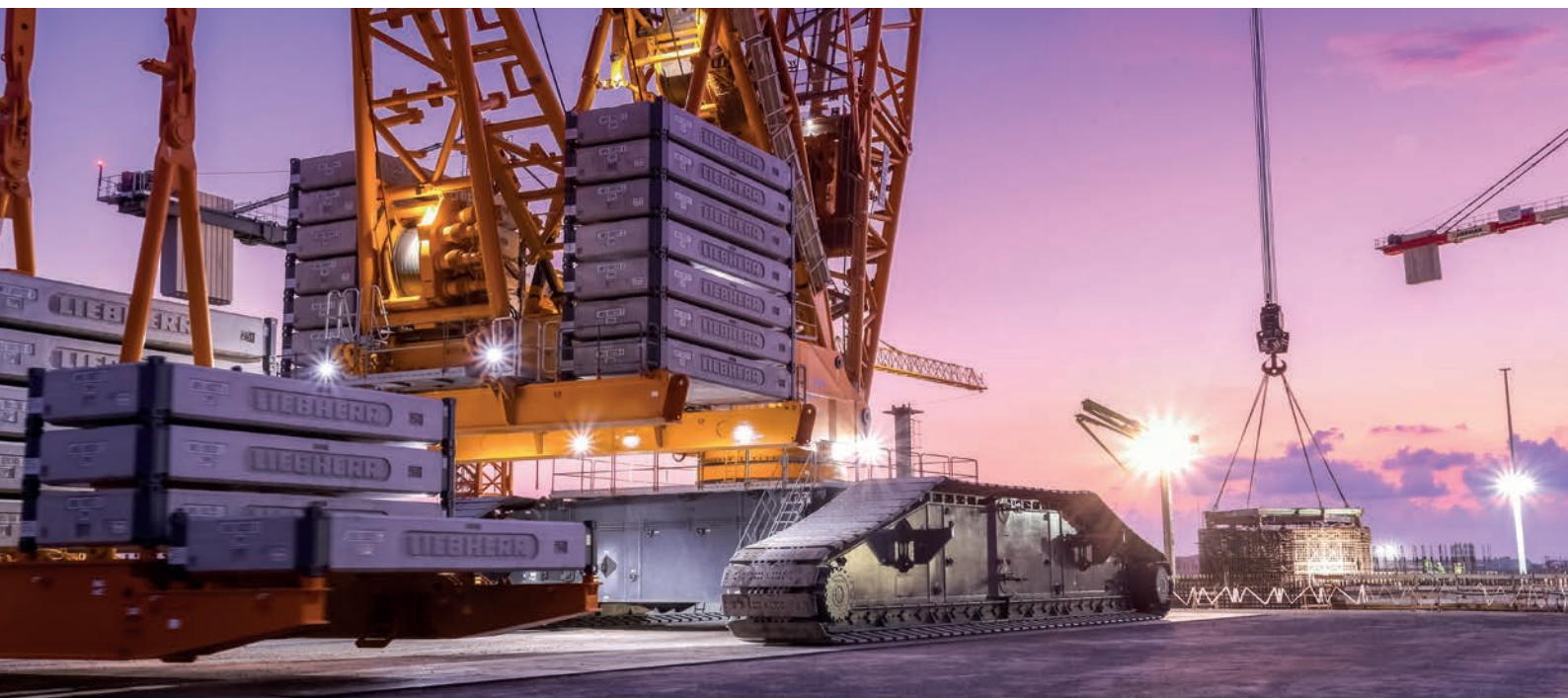
September 2019, Unit 1 reactor cavity conductor installation (Image: Akkuyu image bank, ROSATOM)
