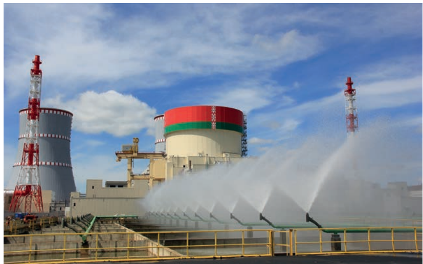
Ostrovets nuclear power plant (Image: ROSATOM)
